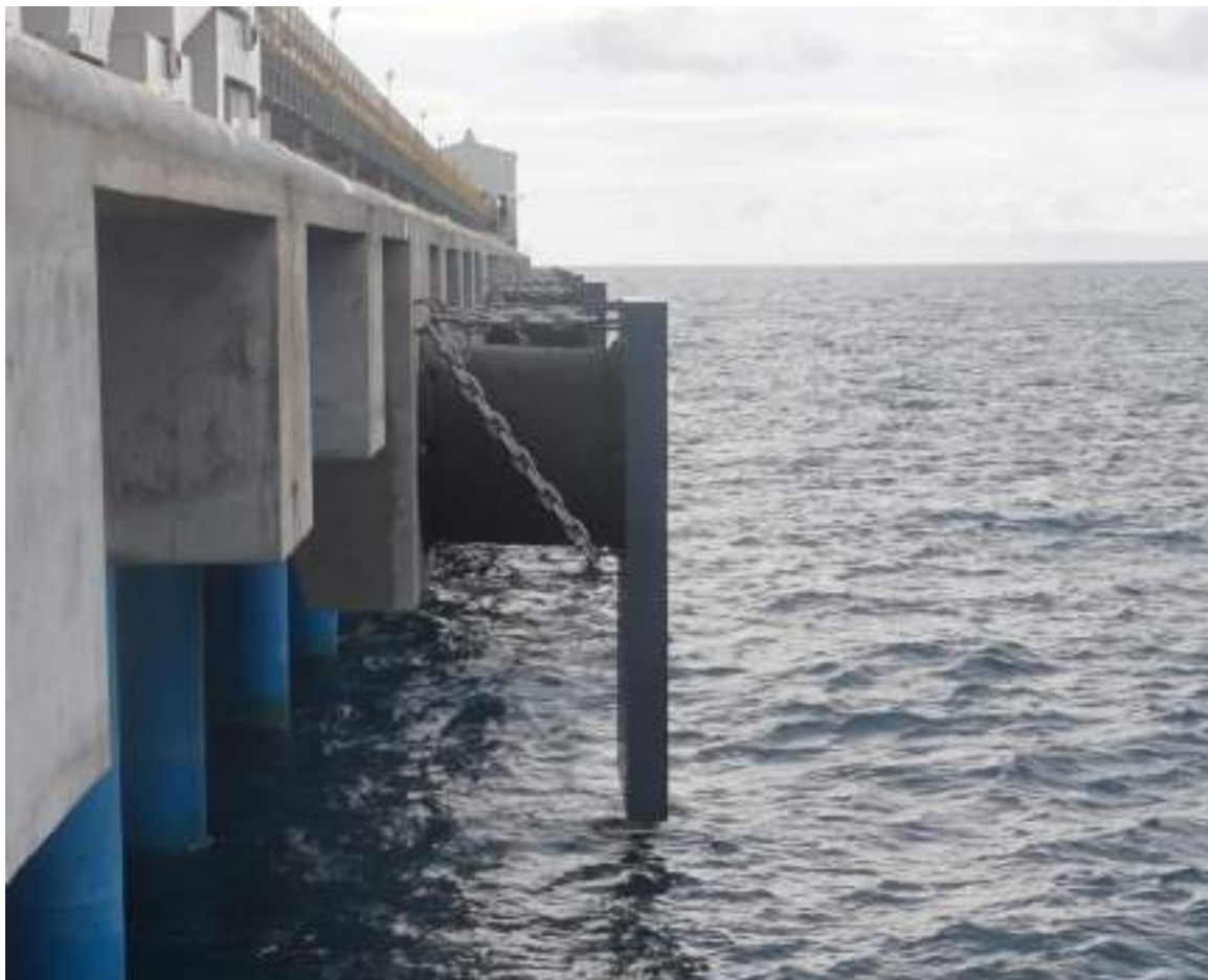
TOLEDO POWER PLANT JETTY, TOLEDO CITY, CEBU HICOR CELL TYPE FENDER
